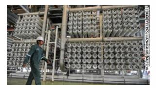
Water is processed through membranes at the NEWater plant to remove solids, microorganisms and other contaminants.
